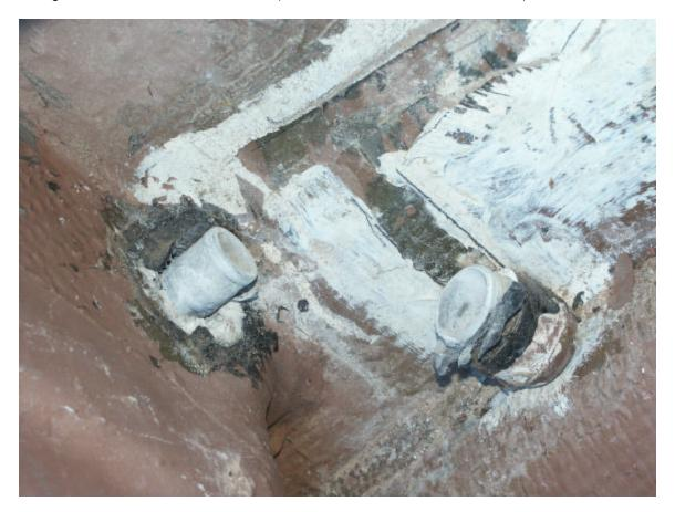
Inside of locker showing pipe from swim step with cap removed on right of picture. Note substantial amount of caulk/sealer, etc.
